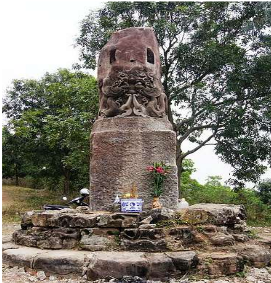
Figure 7: Stone columns at Dam pagoda
